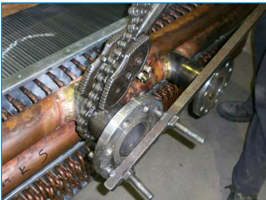
Installing screw-on flange
