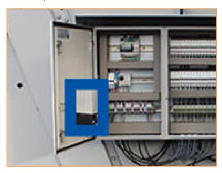
The default electrical panel is equipped to be installed in ambient temperatures that go down to -10°C. For climates where the ambient temperature can become even lower, an electrical heater can prevent damage to the internal components inside the electrical panel for ambient temperatures as low as -40°C.
