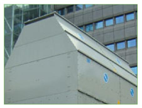
With discharge hoods, you can comply with layout restrictions by **elevating unit** discharge above adjacent walls and increasing discharge air velocity to **reduce the risk of re-circulation** in confined spaces.
