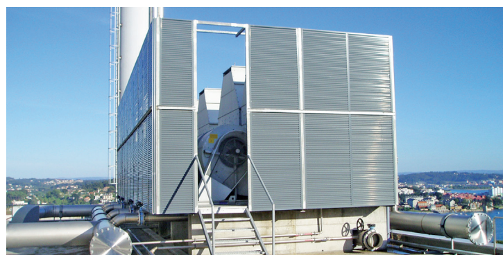
Figure 10: Architectural walls being constructed around Closed Circuit Cooling Towers
