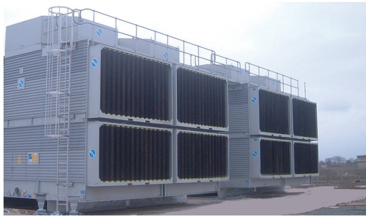
Figure 11: Intake and discharge sound attenuation on a BAC Axial Fan Open Cooling Tower
