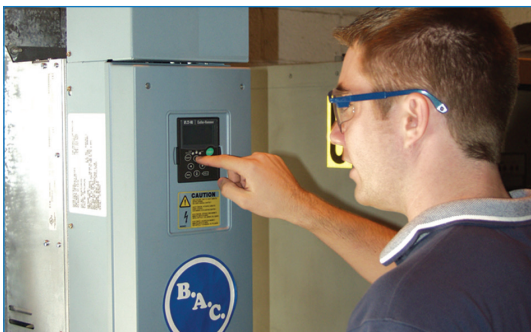
Figure 8: VFD with Integrated Bypass
